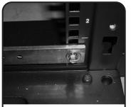
Remove all paint, etc. from mounting surface of cabinet. Remove any oxidation, etc. from back side of the ground bar at the point of attachment to the cabinet using the abrasive cleaning pad. Apply a coating of antioxidant material to the mounting surfaces.
