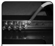
Remove any oxidation, etc. from the mounting surfaces with abrasive pad and apply a coating of antioxidant material. Using (2) of the 12-24 x 1/2" machine screws attach one end of the 96" ground wire to the ground bar.
