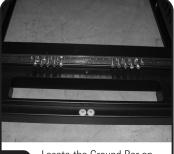
Locate the Ground Bar on the cabinet (the ground bar can be mounted on either the top or the bottom).
