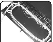
Once cable is secured, termi-12 nate fiber per manufacturer's specifications and route cable slack through fiber management clips. Mate connectors to appropriate adapter and slide tray to the closed position by disengaging the rear latch head.
