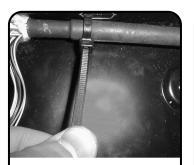
Secure the cable jacket to the tray using a cable tie inserted through the lanced tab formed into the sidewall of the tray.
