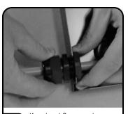
If optional Compression Fitting is used — Use in place of grommet. Position the fitting at least one meter (3.28 ft) from the cut end of cable. Tighten the clamp nut against the cable jacket.
