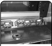
Align flat Quick-Pack latches with the respective cutouts, in the adapter plate bracket and push inward until it snaps into place.
