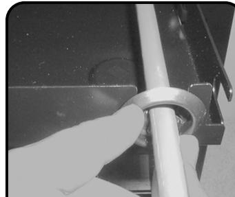
**9** Slide a grommet onto the incoming cable and, to enable sufficient cable slack, push the grommet back one meter (3.28 ft) from the cut end of the cable. Install grommet into desired cable access hole.
