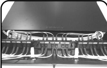
**15** Slide tray out the front (see Step #3) and install jumpers at front of enclosure.
