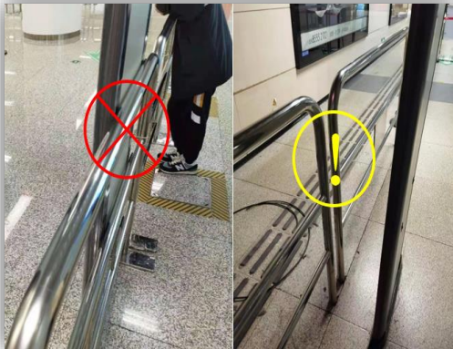
③ WTMD and metal handrail distance \geq 50\text{cm}
