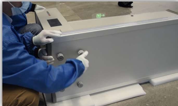
5. Tighten the screws with Allen key
