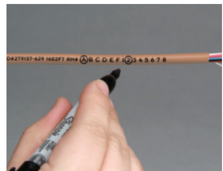
Room and Zone Markings
