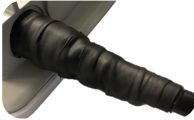
Figure 10-14 Rubber Mastic Tape Wrap around RF Port and Cable/Antenna
