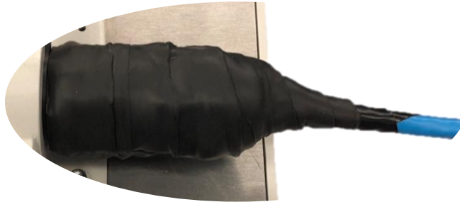
Figure 10-9 Rubber Mastic Tape Wrap around Ethernet Port and Cable
