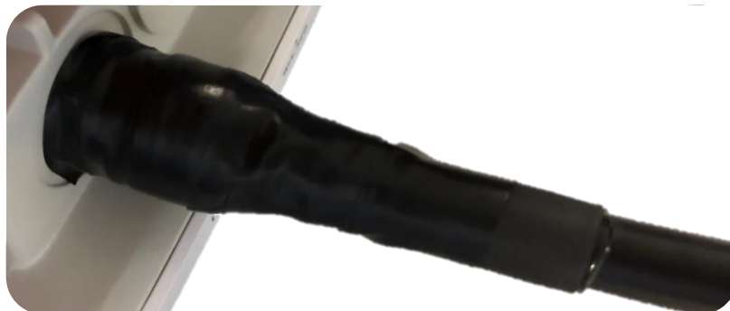
Figure 10-13 Electrical Tape Wrap around RF Port and Cable/Antenna
