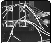
Route the horizontal, or backbone cables inside the S89 bracket and feed the cables out either the right or the left side of the bracket as needed.
