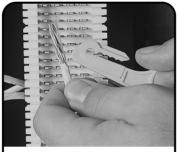
Strip back only as much cable jacket as is necessary to terminate the conductors.
