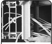
Install the S66 block onto the S89-type bracket.
