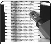
Terminate each conductor using an S814 impact tool or equivalent.
