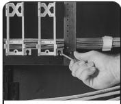
Mount an S89-type bracket firmly on a properly prepared plywood wall using two wood screws; or alternately mount on a Siemon cross-connect frame.
