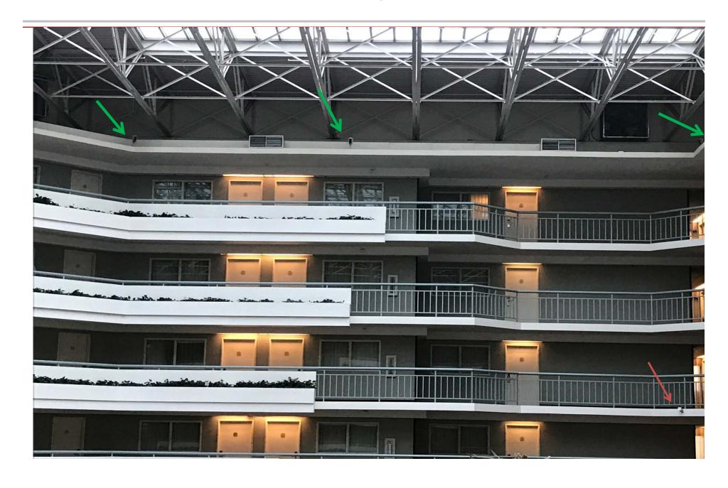
**A.4.5.2** The purpose of using horizontal beams to detect the smoke layer at various levels is to quickly detect the development of a smoke layer at whatever temperature condition exists.
